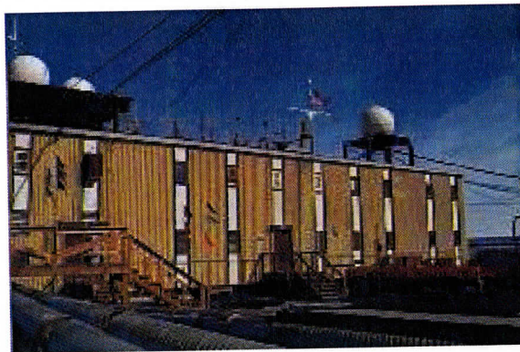
Figure 3 Photo of McMurdo Operations/McMurdo Weather building 165 showing the two Sea Space NOAA and DMSP direct readout reception systems on the left hand side of the building. The system on the right is no longer installed. (Photo courtesy, NSF-OPP)
