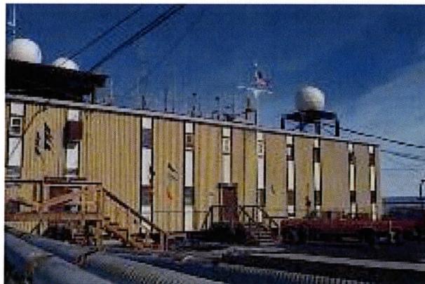
Figure 5 The weather instrumentation shown here atop building 165, McMurdo Operations and McMurdo Weather Office is the source of McMurdo Station's synoptic observations.
