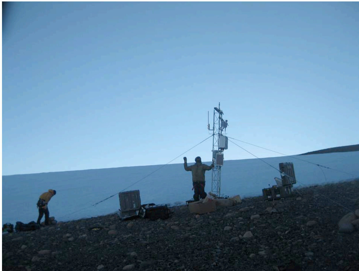
Installation of CR1000 AWS at Evans Knoll on January 12 th , 2011
