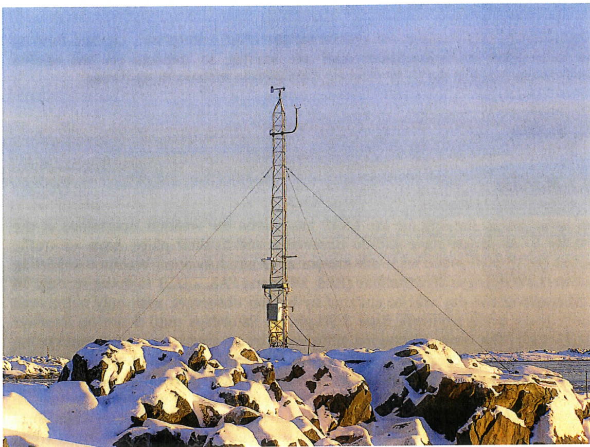
Figure 17. The PALMOS weather observation tower at Gamage Point at Palmer Station. (Photo courtesy of Glenn Grant, ASC/NSF)
