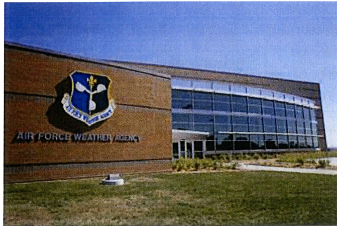
Figure 9. The Lt. Gen. Thomas S. Moorman Building is the headquarters for the Air Force Weather Agency (AFWA) shown here (Photo courtesy U.S. Air Force by Ryan Hansen)
