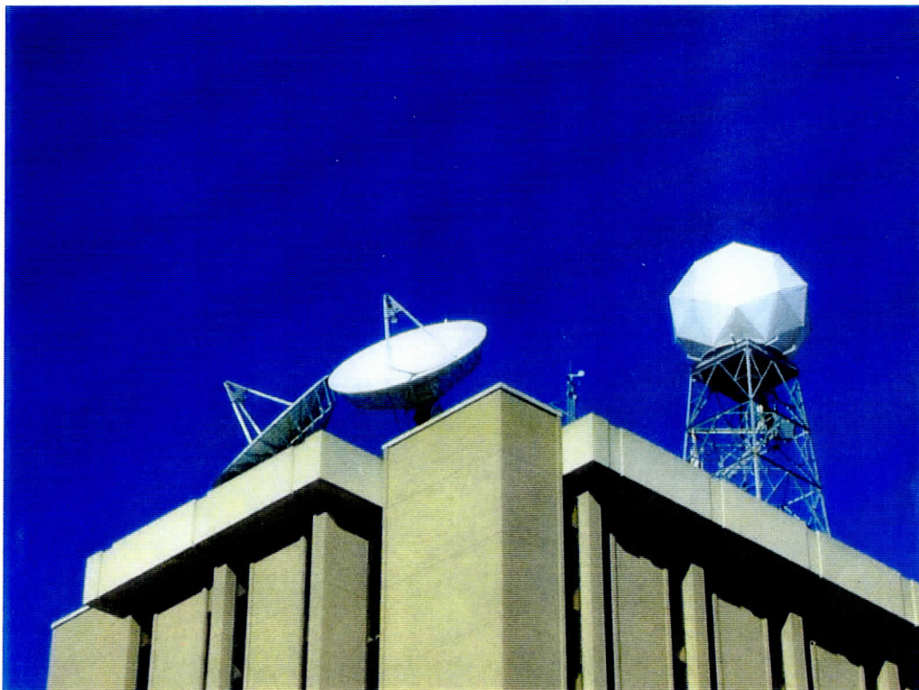
Figure 2: Final location of tower and radome on SSEC roof
