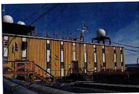
Figure 3 Photo of McMurdo Operations/McMurdo Weather building 165 showing the two Sea Space NOAA and DMSP direct readout reception systems on the left hand side of the building. The system on the right is no longer installed. (Photo courtesy, NSF-OPP)
