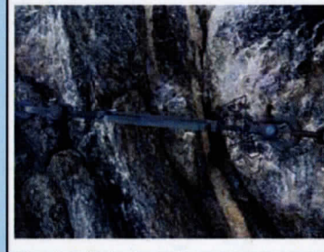
Steel cable tension (Good cond)
