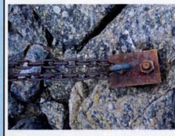
Anchor point (Good cond)
