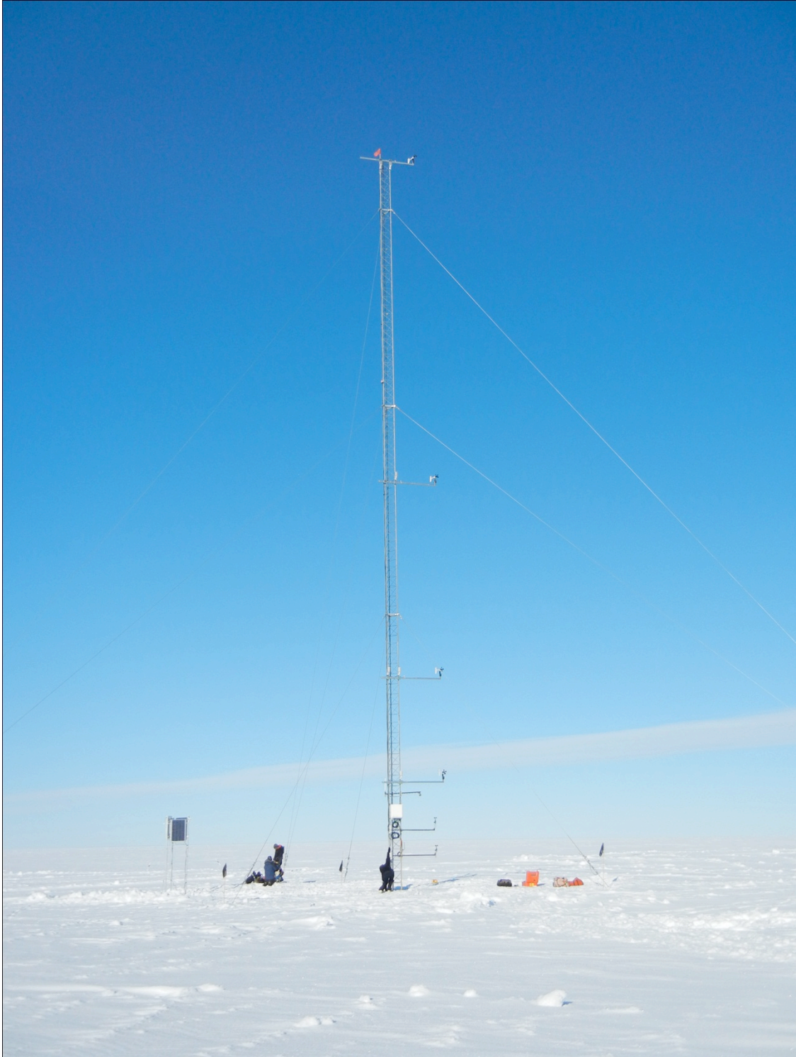
Tall tower after instruments installed on February 3 th , 2011
