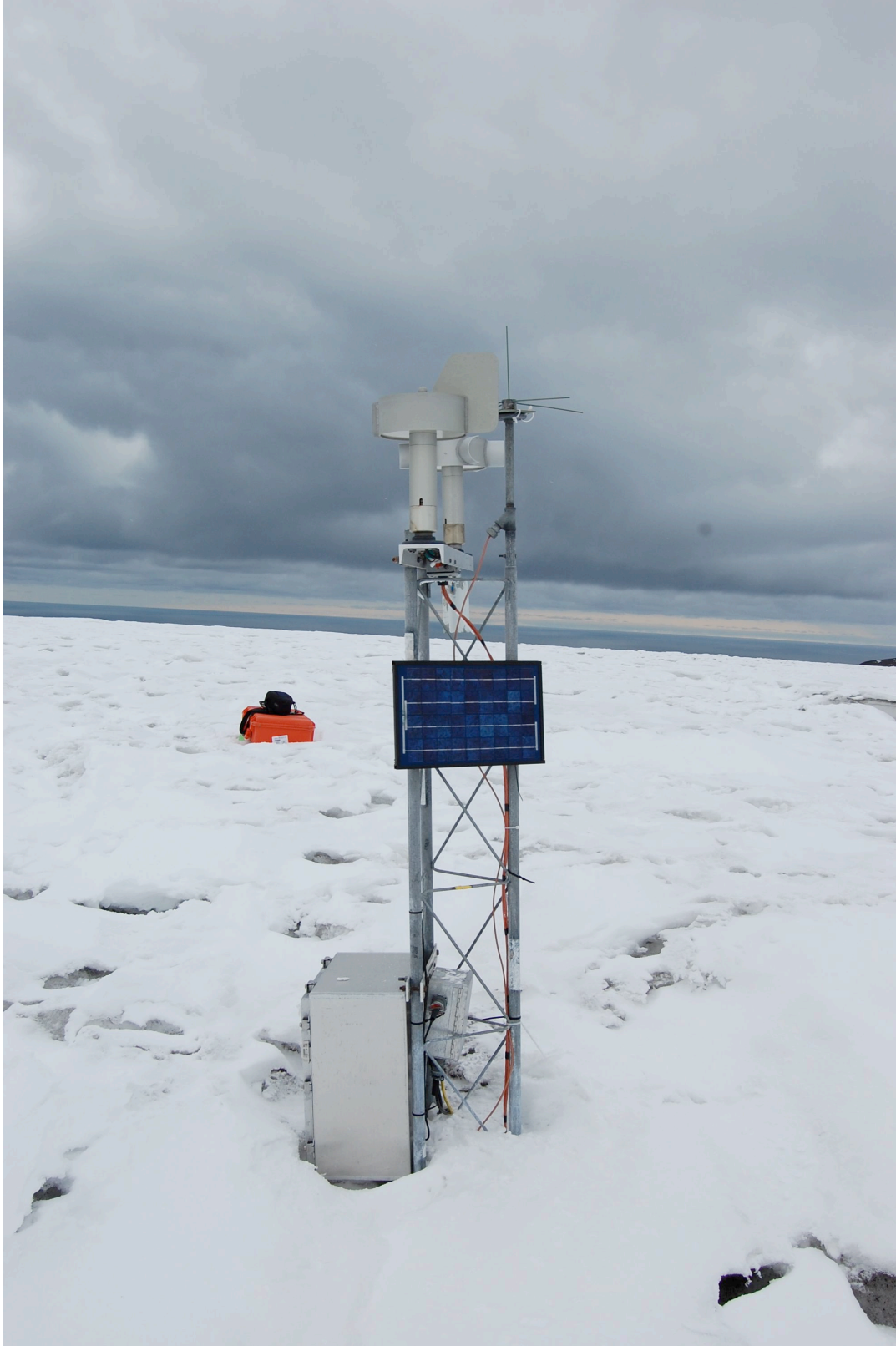
Whitlock AWS2HWS AWS before replacement on January 28 th , 2011
