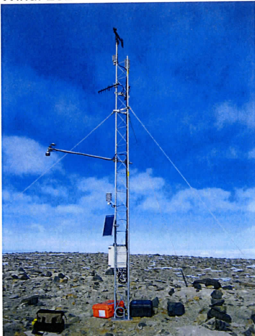
Marble Point II after installation
