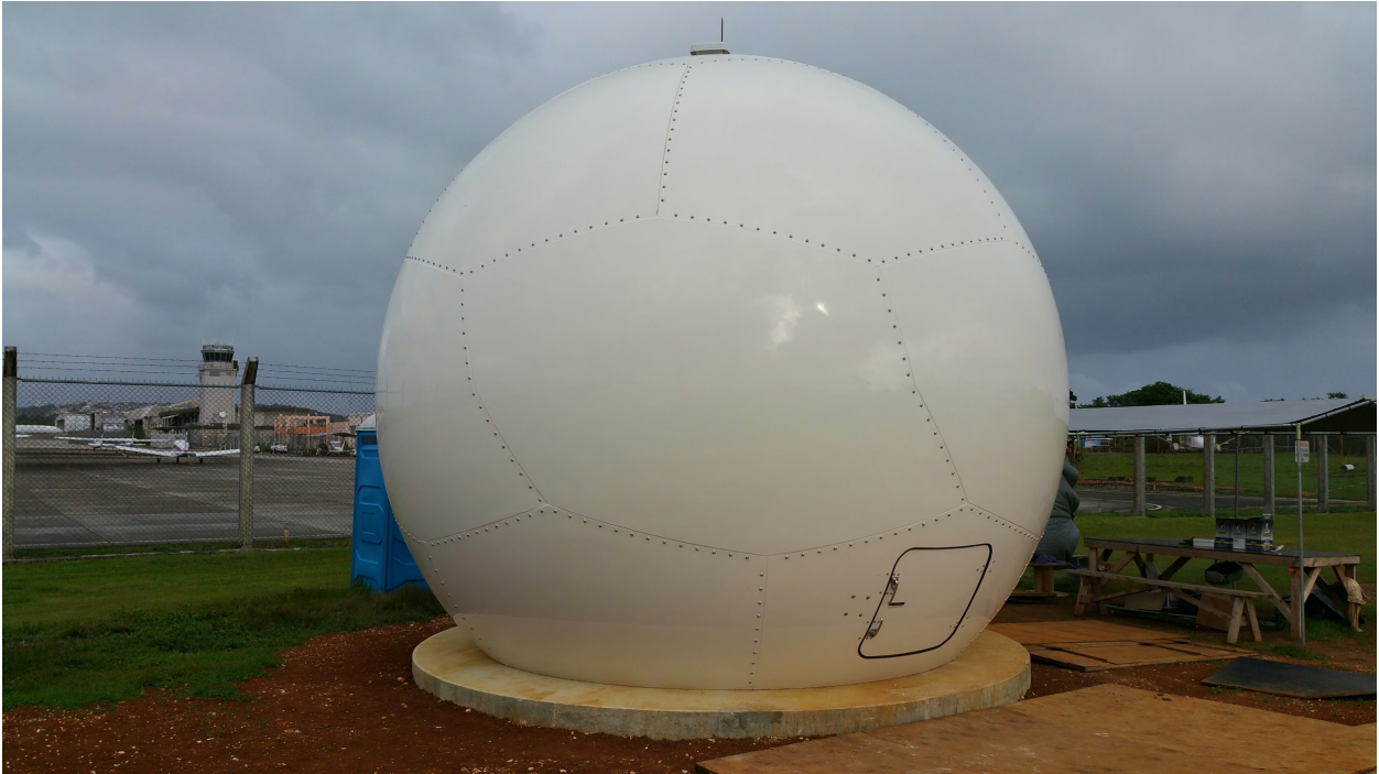
Figure 97. Taken shortly following installation, this photograph shows the radome on the antenna pad. The antenna is inside. The antenna dish is three meters (9.8 feet) wide. The radome is measures approximately 18 feet in diameter, and is capable of withstanding winds up to 190 miles/hour.
